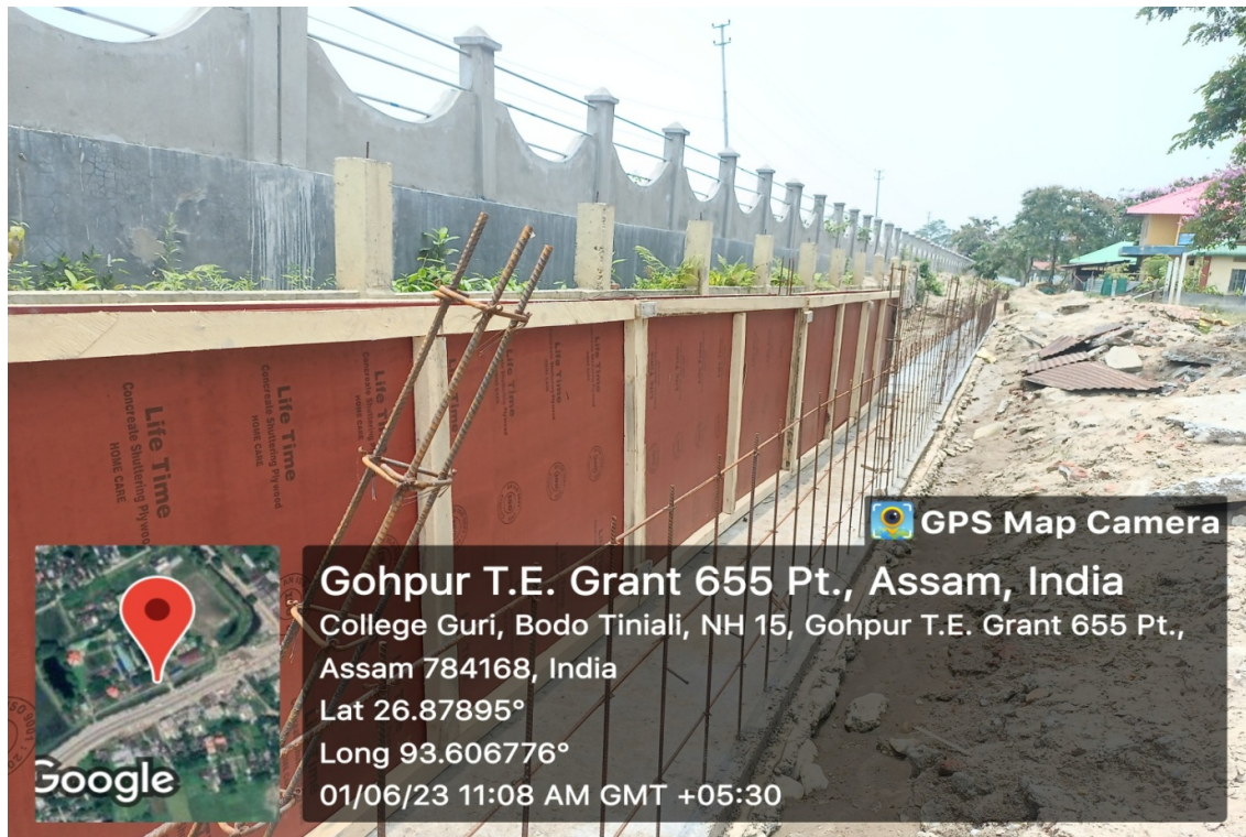
Bunds are constructed
