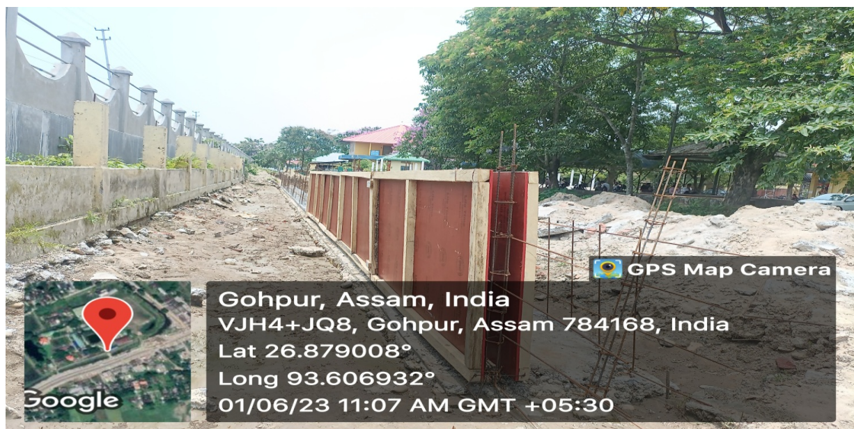
Bunds are Constructed
