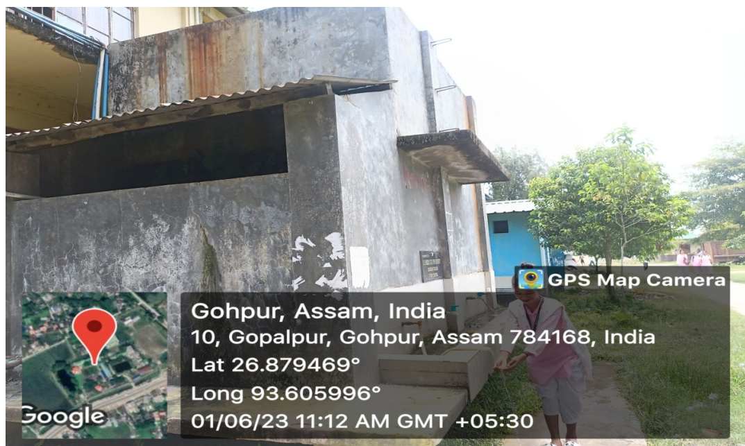
Water Tank and Storage Facility
