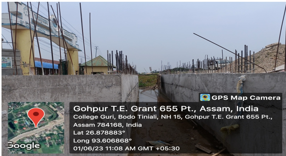
Bunds are constructed
